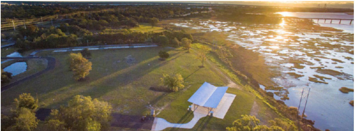
The Bend in North Charleston, South Carolina
