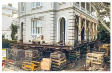
Elevating buildings is one way owners are mitigating stormwater impacts, as seen at 1 Water Street (above, right) and with single houses on Rutledge Avenue (below left) and Savage Street (below).
