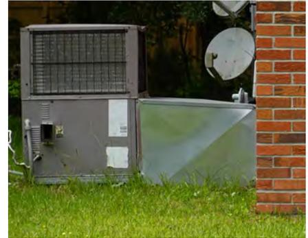
Package-style HVAC systems require more space and exterior ductwork at ground level, which can complicate system elevation. Ducts in flood-prone areas are vulnerable to damage.
