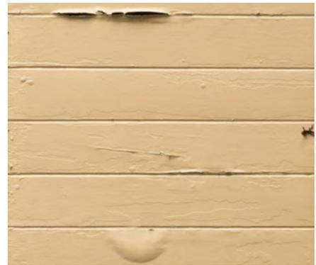
Paint can deteriorate over time or be an indicator of underlying problems that show as wrinkling, peeling, blistering, cracking or crazing, or alligatoring.
