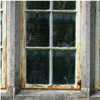
Steel windows can rust, requiring cleaning and rust-inhibitive primer and paint.
