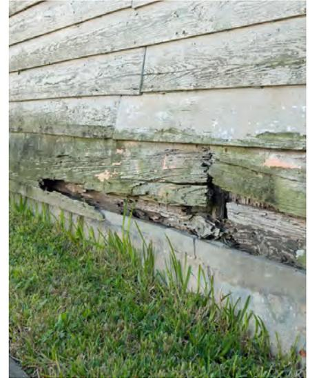
Wood located on or next to a brick or a concrete foundation or pier is more likely to absorb moisture and rot, as well as attract pests and termites. Open joints provide a path for stormwater and floodwater.
