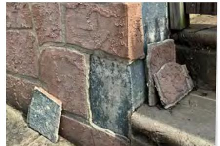
Some newer applications of stucco are intended to look like stone veneer. They are smeared on masonry and not keyed to joints or lath. Un-keyed stucco cracks easily and can peel away from the wall.
