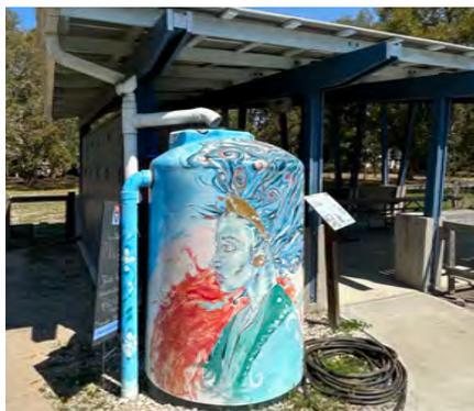
The roof downspout discharges into a rain barrel.
