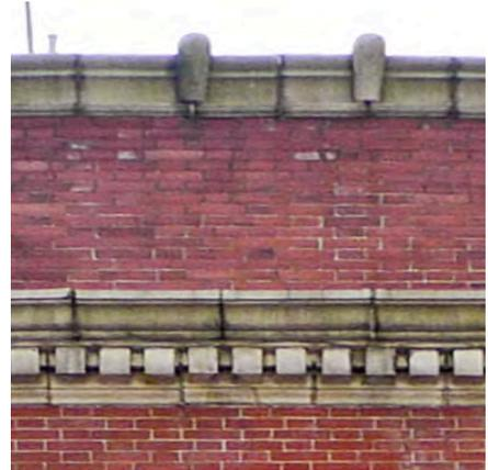
Terra cotta can flake or spall allowing water and wind to penetrate into structural components.
