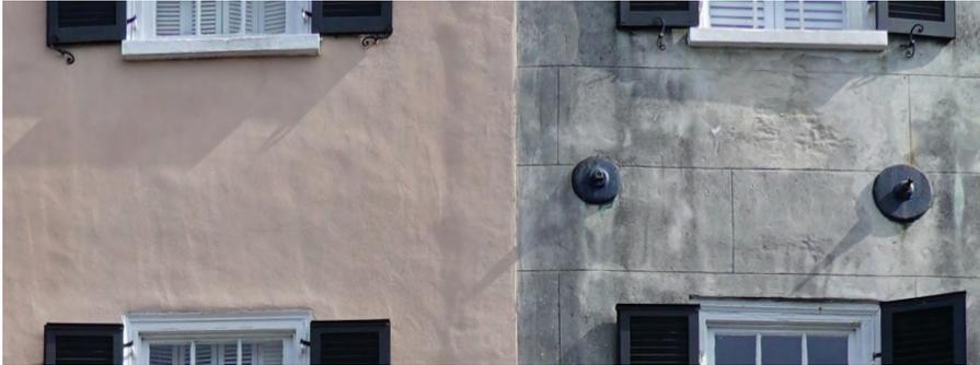
Stucco is a versatile material that can be coated with a color or have a scored finish coat to resemble masonry. It also serves as a protective coating for the underlying masonry or wood structure.
