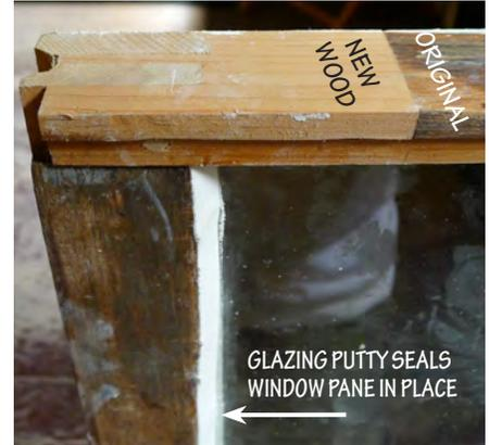
One of the advantages of historic wood windows is repairability. This photograph demonstrates a Dutchman repair at the corner of the historic wood window sash. Also note the application of new glazing putty as part of the repair.
