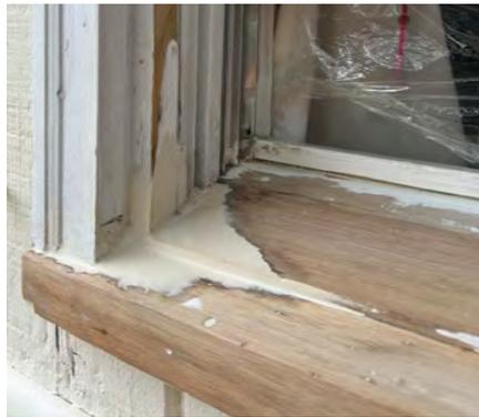
Epoxy has been applied to match the profile of the existing trim.
