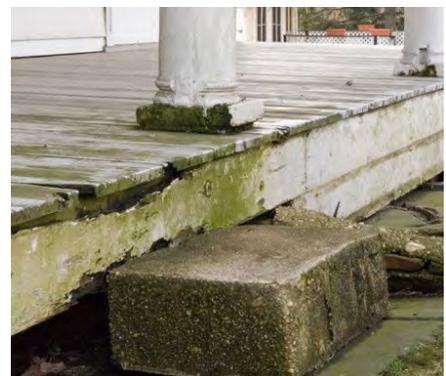
Wood that is in contact with the ground, situated close to plants, or in areas prone to splashing water are particularly vulnerable to rot and must be regularly cleaned and painted.
