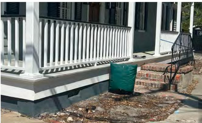
The backflow preventer, disguised by the green cover, keeps floodwater from backing up into drains and plumbing fixtures.
