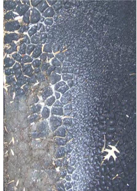
Rubber roofing can crack, eventually forming leaks. Significant cracking of this roof suggests replacement might be prudent. Selecting a lighter color can reduce heat absorption.
