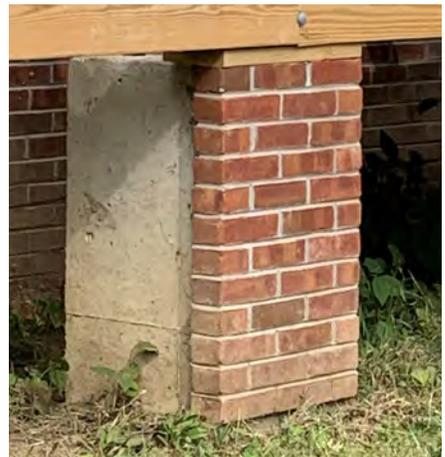
A full-width brick veneer has been installed on this new poured concrete pier at a building elevation to mimic the original appearance.
