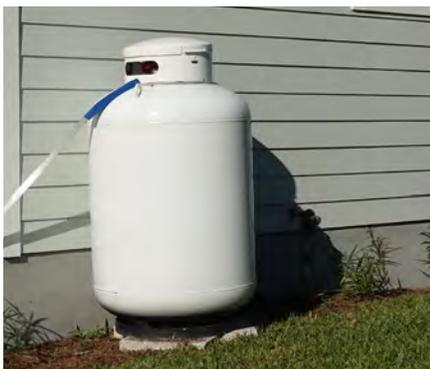
Secure propane tanks to reduce movement during a flood or earthquake.
