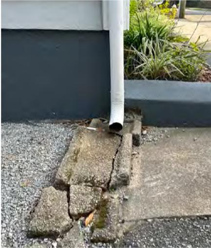
Avoid locating downspout discharges near masonry walls and foundations.
