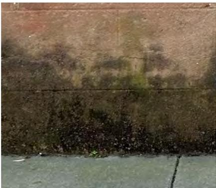
The algae along the foundation suggests significant moisture in the wall. Possible sources can be pooling adjacent to the wall, rising damp, or rainwater splashing from the sidewalk.
