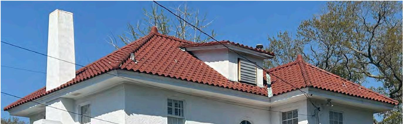
The roof eave projects beyond the building wall below. Eaves can be open, with exposed rafter tails, or boxed with vented spaces (as in this example).
