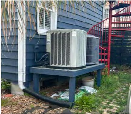
Stands for elevating equipment can be purchased or made from lumber at home. Stainless steel or galvanized connectors will limit rusting.
