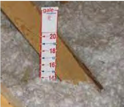
Loose insulation should be measured to monitor depth. (energy.gov)
