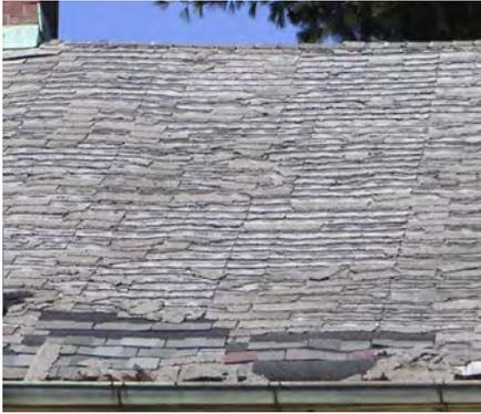
Individual shingles are missing and others are in a deteriorated condition.
