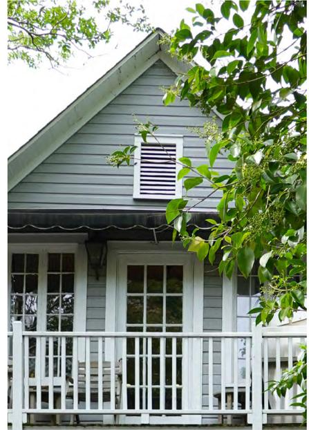
Any openings, including attic vents, will need temporary storm protection.
