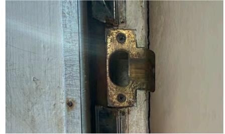
*Throw-plates should be well secured to prevent doors from blowing open.*
