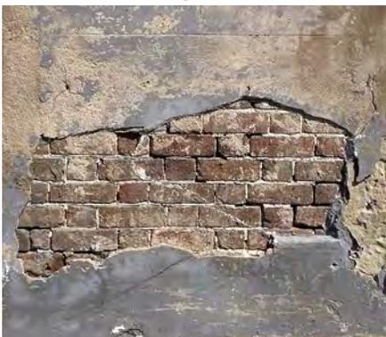
The loss of a stucco coating from a masonry wall can allow water to be absorbed by the underlying masonry, advancing deterioration of the brick and mortar joints.
