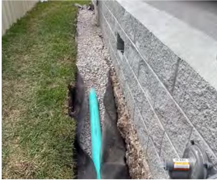
A French drain collects and moves water away from the foundation to reduce building water damage. (LSU Ag Center)
