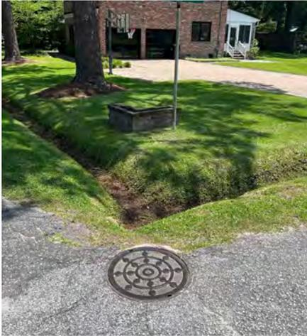
Connected ditches (**bioswales**) collect stormwater from roadways and properties, allowing it to absorb into the ground. Water tolerant plantings can be added, similar to a rain garden. (Refer to Rain Gardens, page R2.6.)
