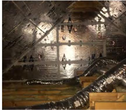
Relocate ducts to attic, above potential floodwater. Installing new insulated ductwork will increase system efficiency. ([www.energy.gov](http://www.energy.gov))
