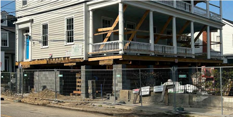
Concrete blocks are structural masonry units typically covered in stucco or a masonry veneer, or painted. Reinforced blocks have poured concrete and steel rods connecting the individual units and is an approved foundation material for building elevations.
