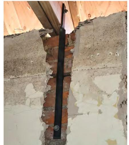
A structural engineer or architect should select and design the hurricane-rated connector layout best suited for the building conditions. The installation requires access to structural elements, like masonry walls and wood framing, necessitating removal of interior finishes.
