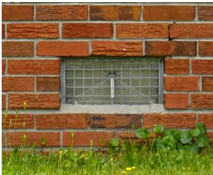
Flood vents may be installed new, or in existing openings in a foundation if they meet design and spacing requirements.
