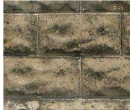
These cast stone blocks are made of concrete and formed to appear like stone.
