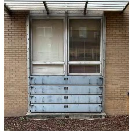
Engineered barriers can include metal panels installed in jamb channels to a height above anticipated floodwater. They typically provide greater protection but are more costly than pre-manufactured options.
