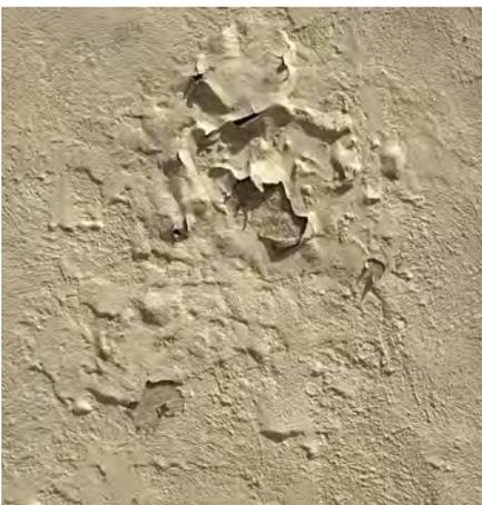
Moisture trapped in the wall is causing the acrylic paint to fail. Complete paint removal and application of a breathable coating may be required.
