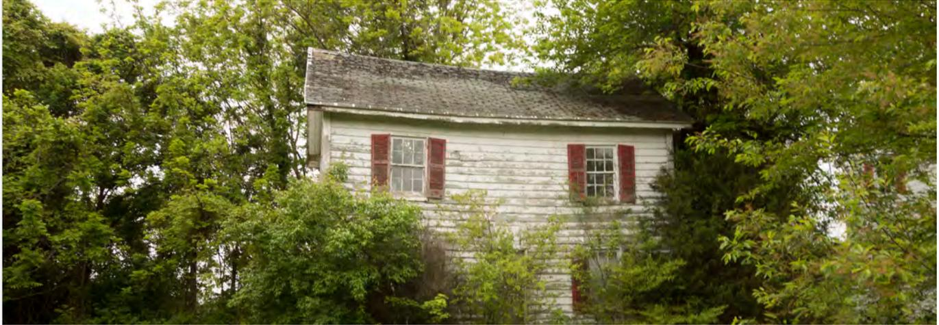
*This roof needs shingle replacement and evaluation for structural repair. Overhead trees limbs should be trimmed so they are not touching the roof.*
