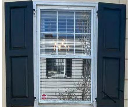
Storm windows with tempered glass or impact-resistant glazing provide protection from windborne debris. (Not approved on historic properties.)
