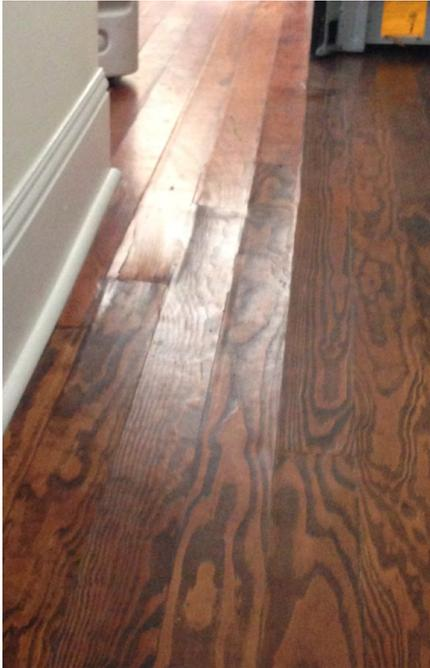
Wood floors can 'cup' while curing and should be dried out slowly after a flood.
