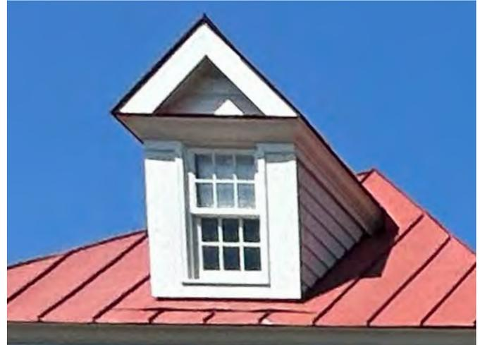
Dormer windows have flashing at the top edge, along the roof slope, and below the window.
