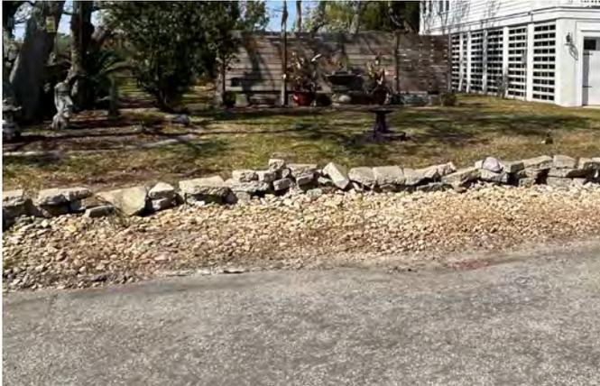
Identifying problem areas can help the design of solutions to guide water flow. The quantity of roadway stormwater runoff reaching the lawn is reduced by absorption through the gravel bed. The larger stones contain the gravel to minimize spread. Installing a smaller gravel bed may be a task that can be completed by property owner. Specialty equipment can be rented or a contractor hired for larger areas.
