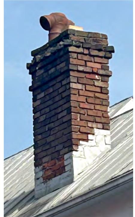
*Mortar joints between bricks may need to be repaired to prevent weak spots and potential structural failure. Stepped flashing is found at the base of the chimney along the roof slope.*
