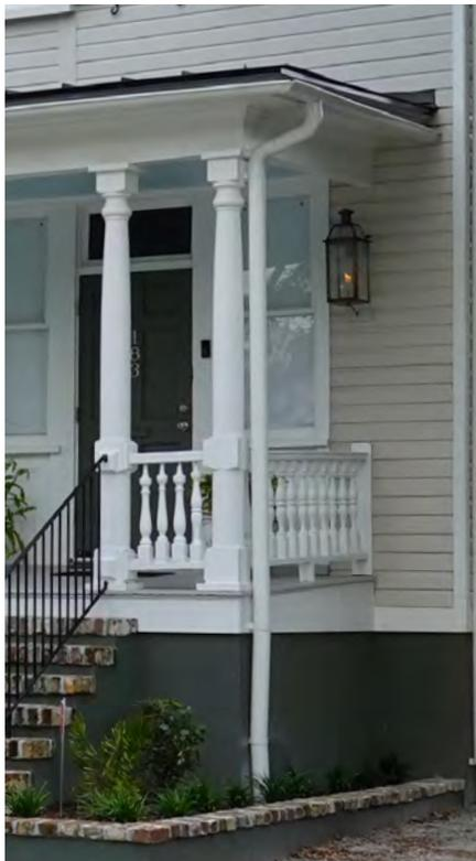
A system of gutters and downspouts can direct rainwater away from the building if kept clear of debris.
