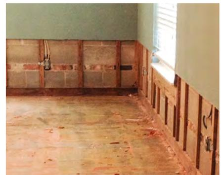
It is easier to relocate electric outlets to reduce future flood damage when wall finishes are removed and repaired.
