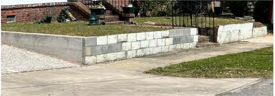
**Grading** refers to leveling an area or changing the slope to control water flow. A retaining wall maintains soil height above the street level, which is lower along the sidewalk.
