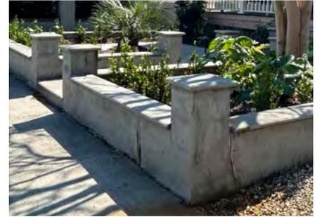
Low retaining walls can be used to manage a change in slope, control water flow, and collect stormwater to allow it to percolate.
