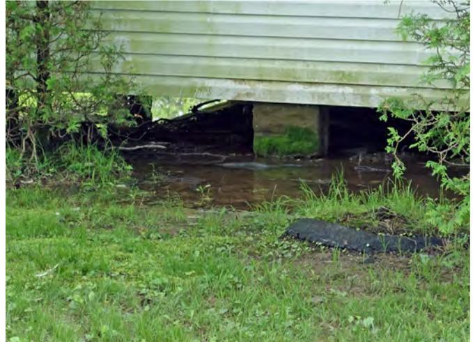
Water is pooling under this building. Prolonged exposure to standing water can compromise the mortar at the cast stone piers, making the building more vulnerable to damage from flooding and earthquakes. Ways to divert the water away from the foundation should be evaluated.
